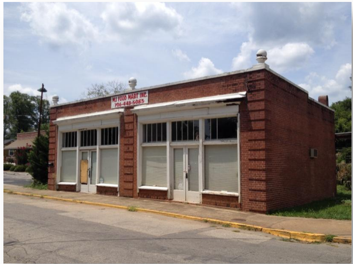
Figure 9: Hillside neighborhood center commercial structure.
