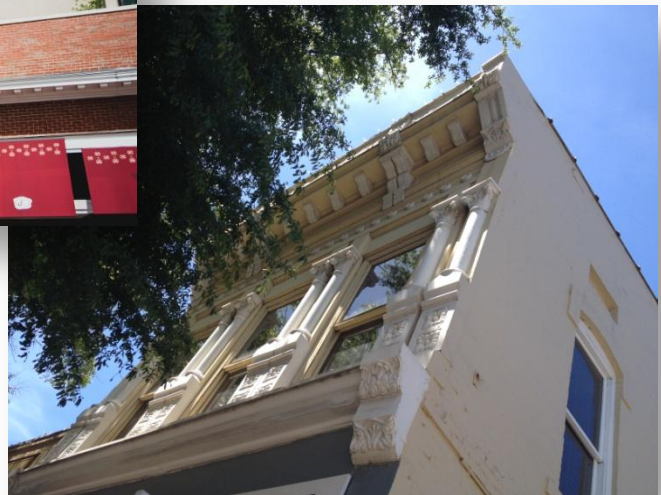
Figure 3: Downtown building containing historic metal facade.
