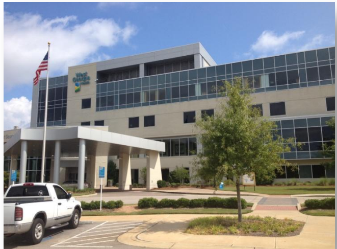
Figure 17: West Georgia Medical Center
